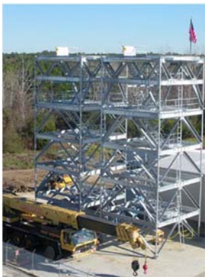
AN/TPS-75 D3 55' Air search radar tower/platform
