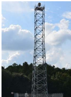
Ground Based Sense and Avoid (GBSAA) radar towers (up to 150')
